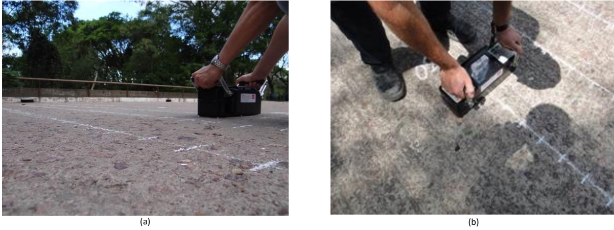
Figure 2. (a) and (b) 3D Tomography to evaluate a bridge deck.
