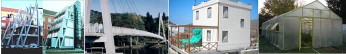
Figure 1. Structures built with GFRP profiles.
