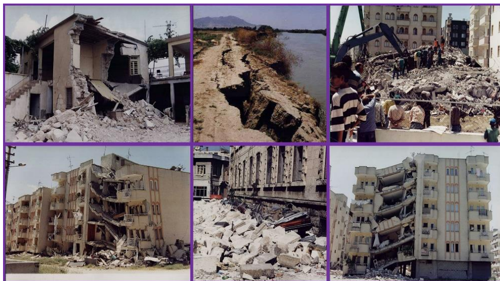
Figure 2. Examples of structures damaged in the 1998 Adana-Ceyhan earthquake (DEMA).
