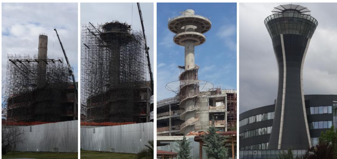
Figure 2. Construction progress of UOT.
